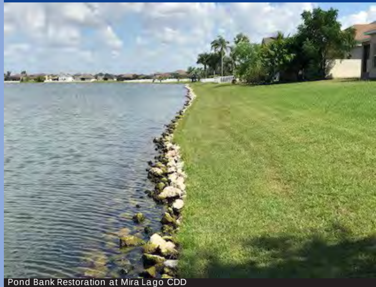
Pond Bank Restoration at Mira Lago CDD
