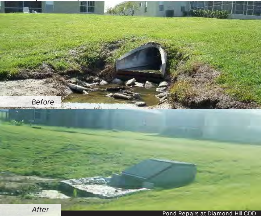
Pond Repairs at Diamond Hill CDD
